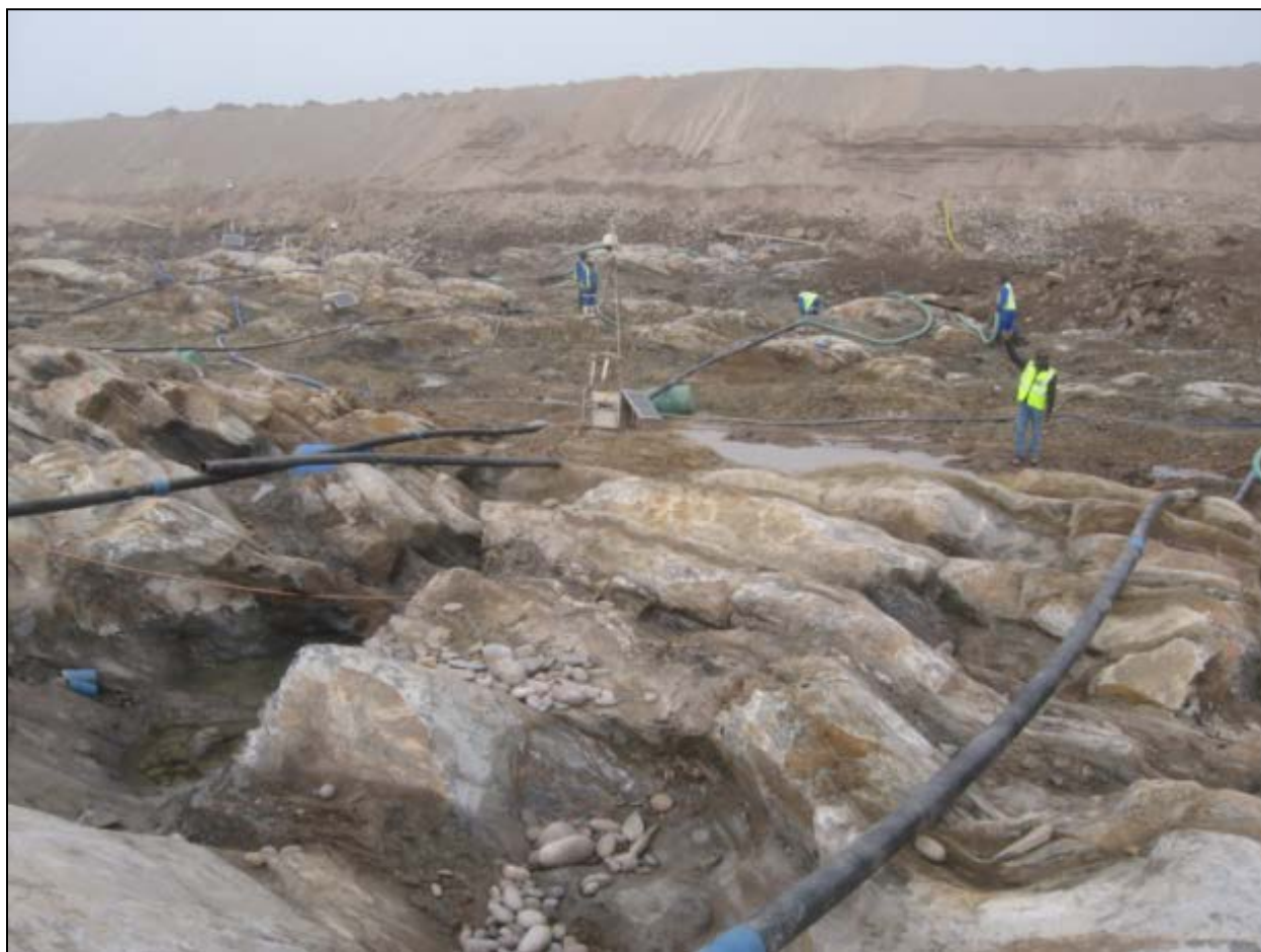
Bedrock cleaning operations – Mining Area No. 1
