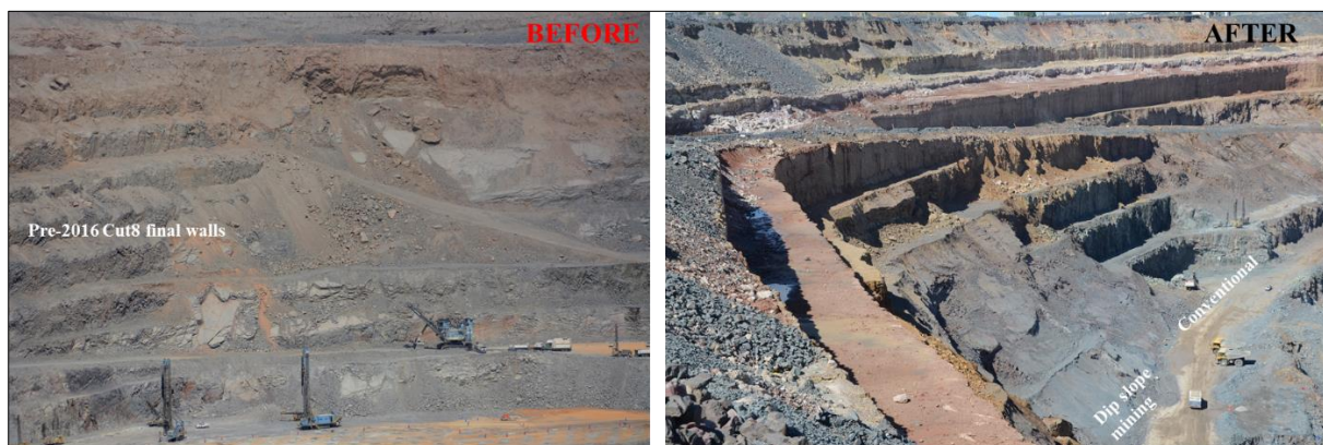
Figure 5: Pit wall conditions before and after implementation of dip slope mining
